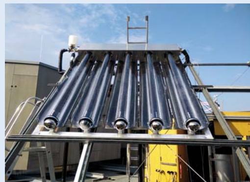
Fig. 5: Picture of the installed sorption collector prototype on the roof of the laboratory in Gleisdorf, Austria
